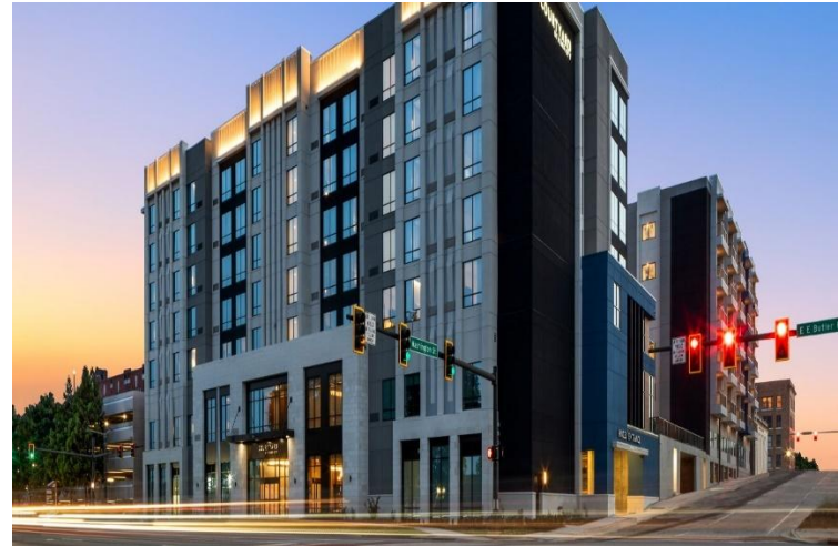
Figure 5: Preferred architectural style for proposed Downtown Monroe Hotel - Courtyard by Marriott in Downtown Gainesville, Georgia (building height limitations may apply).
